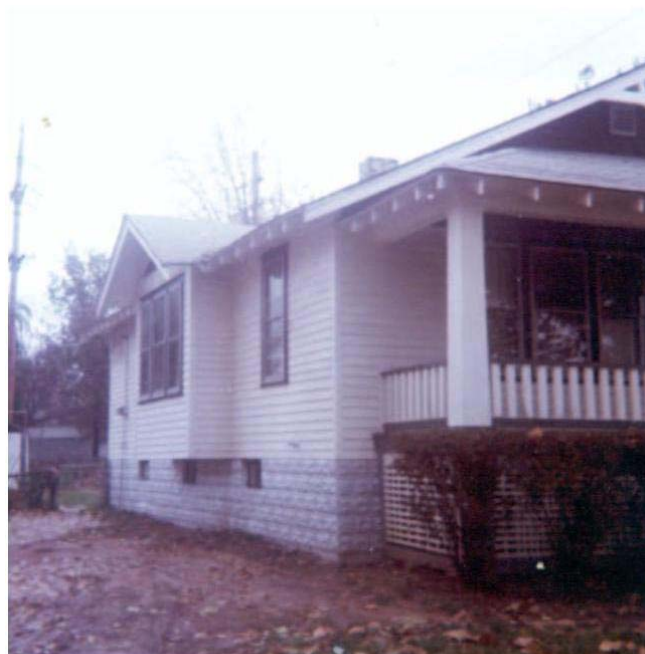
North side of 614 North 82nd Street, East Saint Louis, East Saint Louis Township, Saint Clair County, Illinois posted by Bonnie Kathleen (BACH) Pratt
